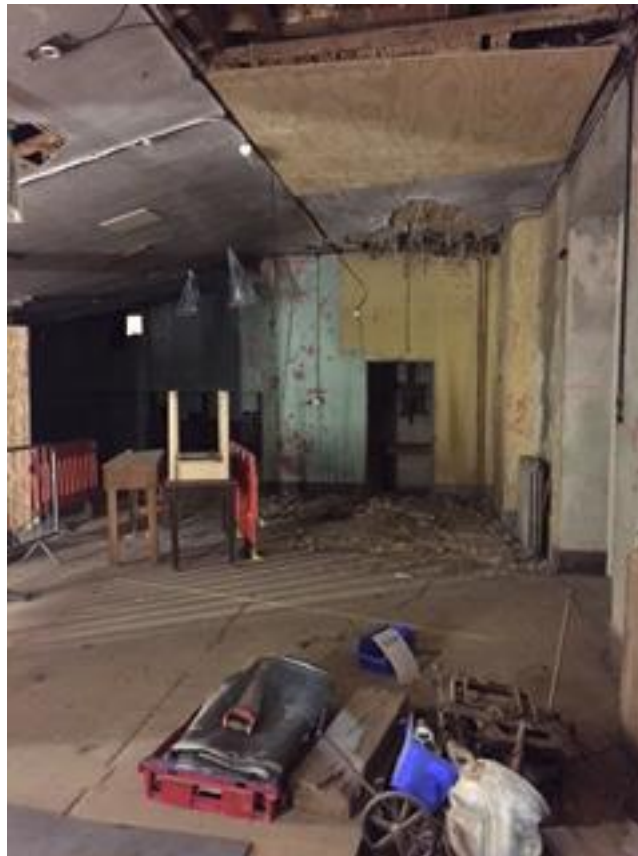
Image of under the theatre balcony
