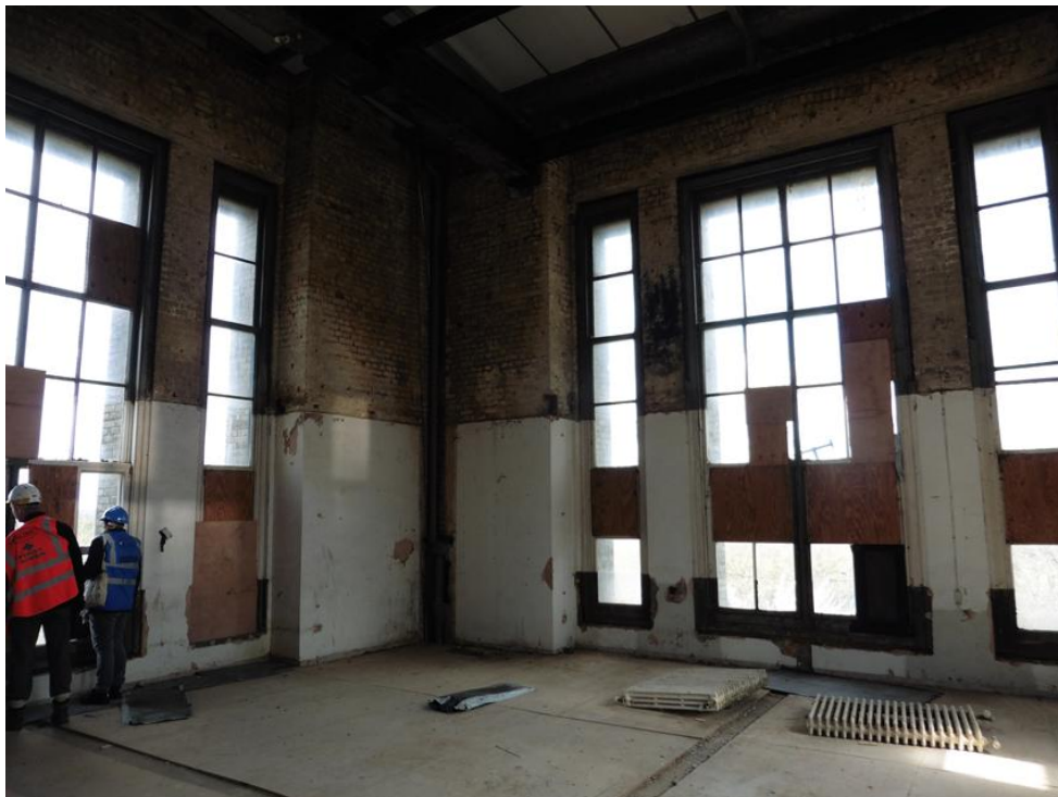
Image of the South East Tower First Floor
