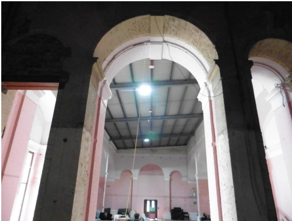
Image of the far arches open and the 1980's ceiling removed in the theatre foyer
